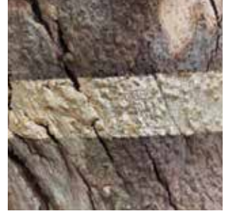
27 ROBYN VENEER SWEENEY Containment Lines NSW
